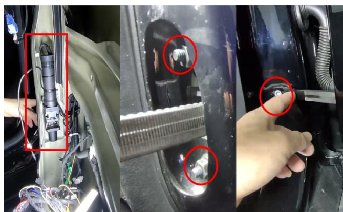
6. 拆下原车限位器安装智能门执行器 Remove the original stopper , and then install our intelligent actuator.
