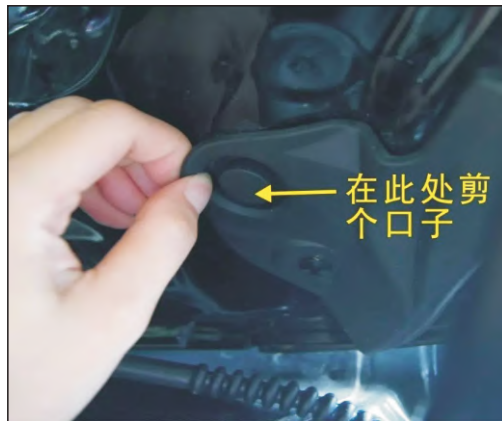
4. Remove the stopper is cut open a vent, conducive to hall wire threading (left and right side steps)
