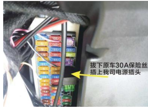
3. Connect power and ground under the driver compartment
