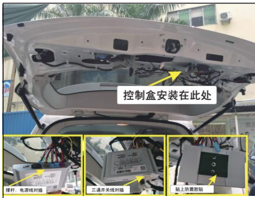
14. Installation of ECU Control Box Insert the plugs into the corresponding socket according to the color and shape (check whether the socket is tightened or not)
