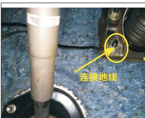
5. Found at the bottom of the main driving ground, ground connection
